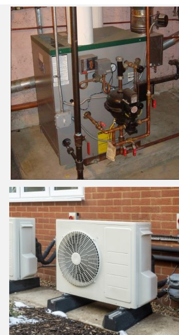
Figure 2: typical natural gas boiler (top) and typical ductless air source electric heat pump (bottom). (U.S. DOE)
